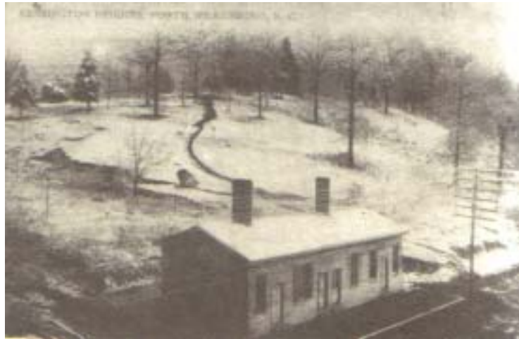
Photo of the North Wilkesboro Train Depot on Kensington Heights. Circa 1890's.
